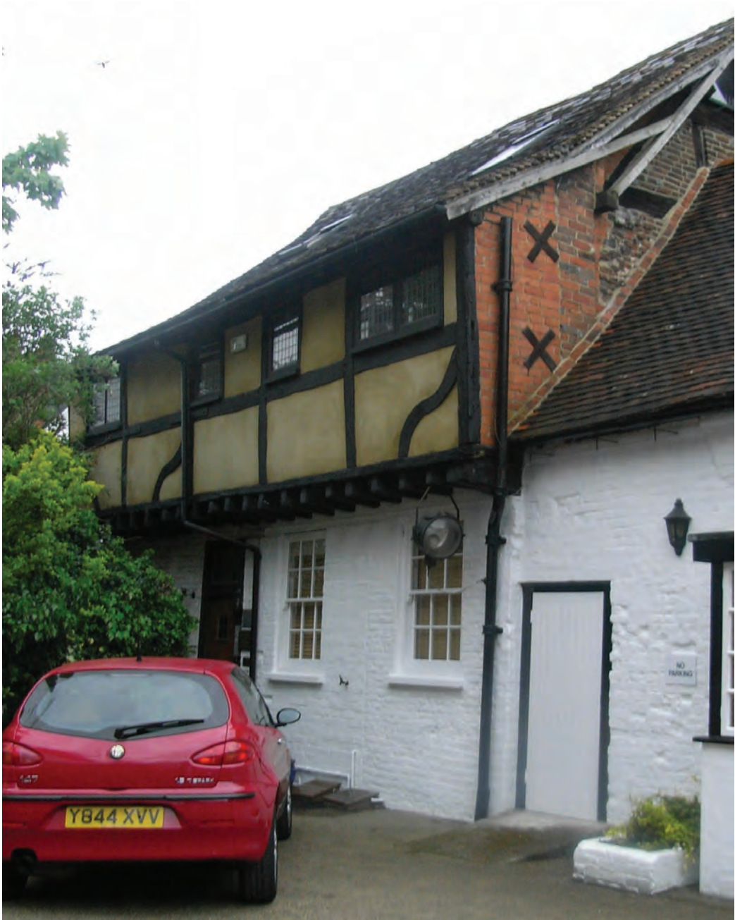
Plate 4. Surviving medieval building at the rear of the White Hart, Henley, with the single-storey former stable block on the right. Photograph by Vic Allison. [Allison, p. 71]
