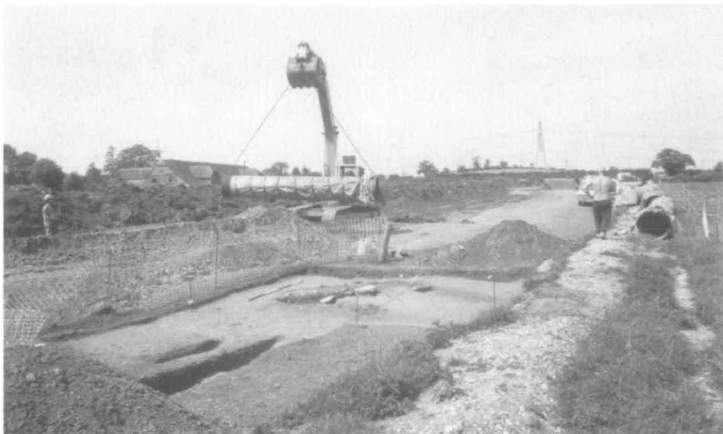
Fig. 17. Lower Farm, Nuneham Courtenay: view of the excavations from the S.E., with the pipes being laid; Area 2 is in the foreground.
