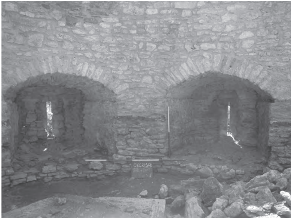
Fig. 6. The unblocked embrasures 1 and 2 within the bastion.
